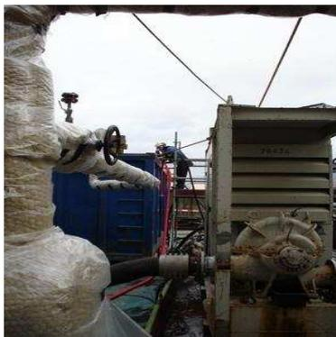
Prior to cleaning, a laboratory examination is carried out so that the method and the cleaning agents required could be determined. The chemical cleaning is carried out following the traditional method: degreasing (for instance with Careclean Degreaser HD), pickling (with Careclean Pickling Liquid) and passivating (with Careclean Passivation Liquid CA)
